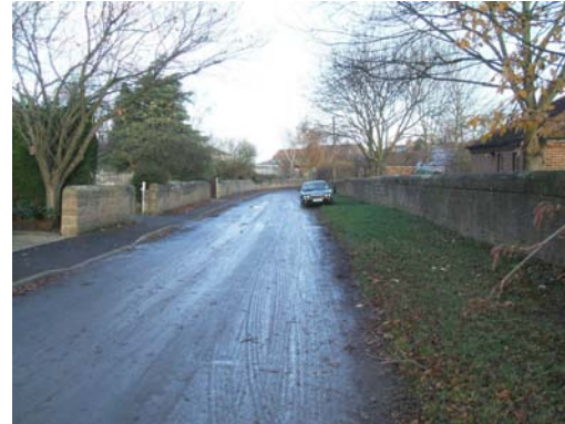
Sandstone walls at the eastern end of Church Street.
