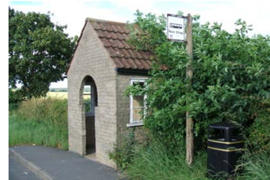
Bus shelter on Station Road with the 'softening' effect of planting.
