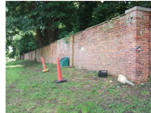
The Park wall along Church Street.
