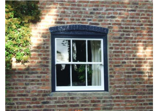
Vertical Sliding Sash window in Post Office Cottage.
